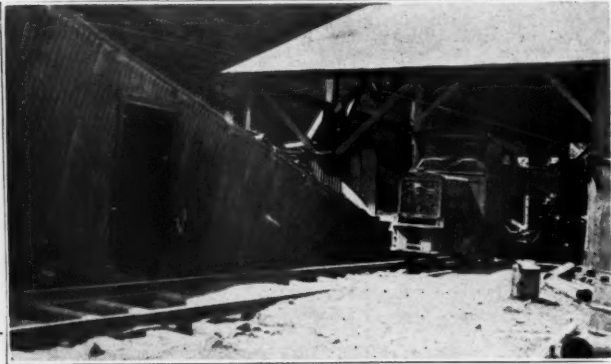
Delivering Stone at Primary Crusher
